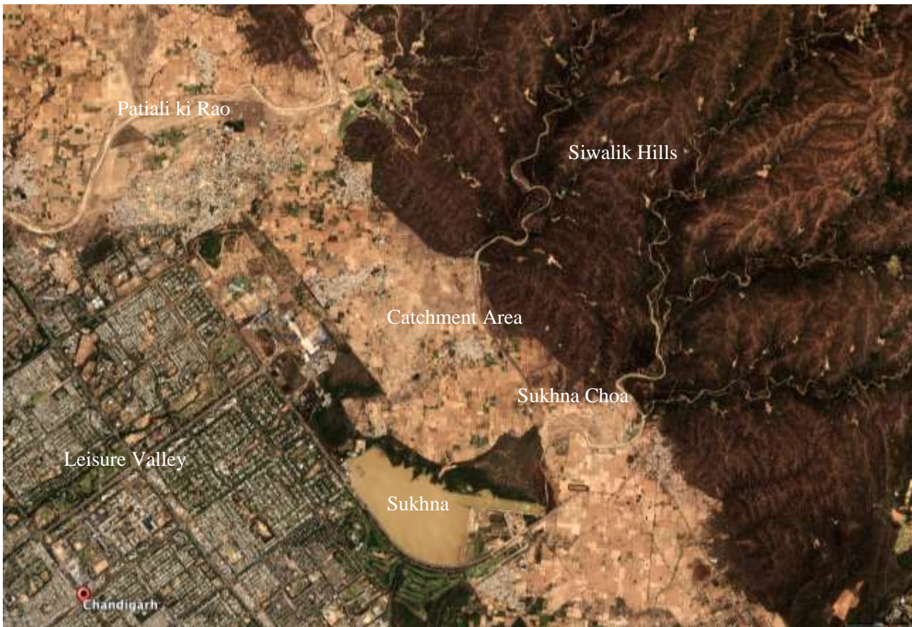
Map 06(a): Satellite Image of Northern part of Chandigarh in 2002 (Source: Google Earth)
