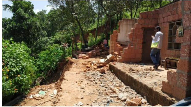
Fig 1.3 Land slip occurred can be seen on slope behind the damaged house
