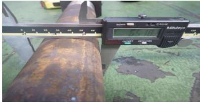
Figure 3. Outer diameter measurement on anchor bolt
