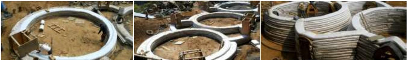
Figure (9) group of photos for the progress in walls build up using earthbags technique (Author 2016, project in Egypt)
