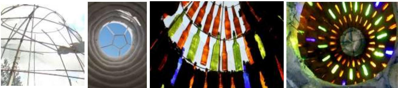
Figure (10) group of photos for the progress in ceiling build up using earthbags and glass bottle technique (Author 2016, project in Egypt)
