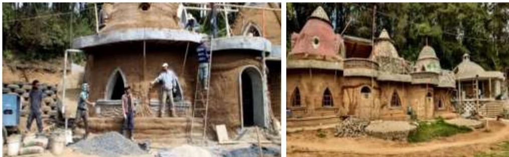
Figure (13) shows the finishing works for the complete unit. (Dabaieh, M., 2012)17
