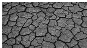
Figure 1.1 Black Cotton Soil in Dry Condition Cracks
